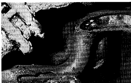
Photo. 1. Melted piping of Q-BOP bottom after back-fire trouble.
