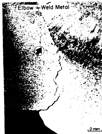
Photo.1 Cracks detected in circumferential weld of elbow (20B) and pipe
