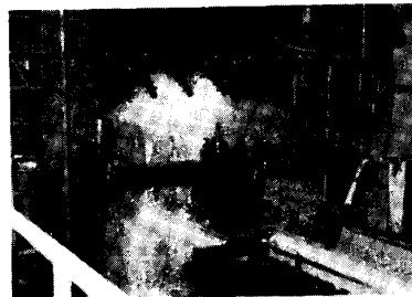
Photo.1 Operation of airless mist cooling
