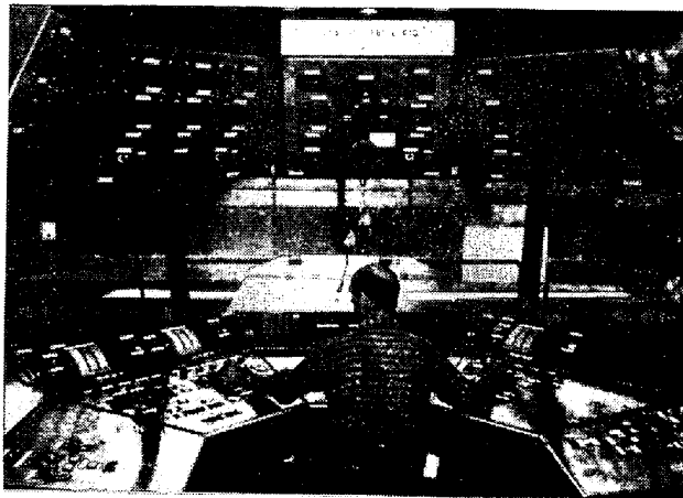
Photo. 7. Wide strip mill control room.
