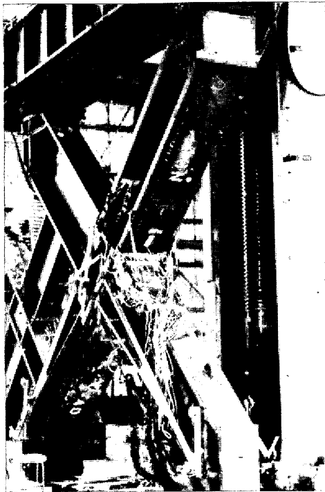
Fig. 11. Test of X type full-size beam-to-column connection. Top right to bottom left is column and top left to bottom right is beam. Loading girder is shown in upper part.
