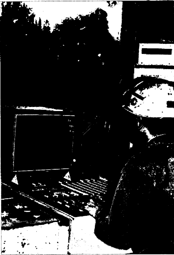
Photo. 1. CRT and pulpit input station in the operating room.
