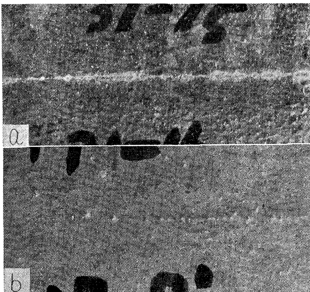
Photo. 1. Macroscopic observations of seamy defects on galvanized steels.
