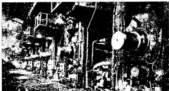
Photo. 1. Tandem hot strip mill.
